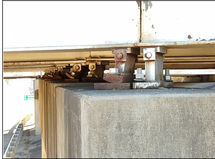
Span 2 bent 2 rocker bearings
