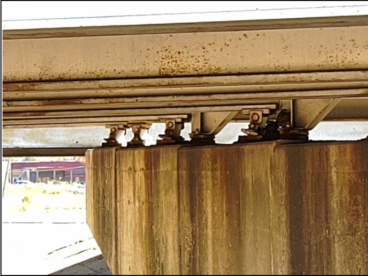
Span 2 bent 2 rocker bearings 3 - 6
