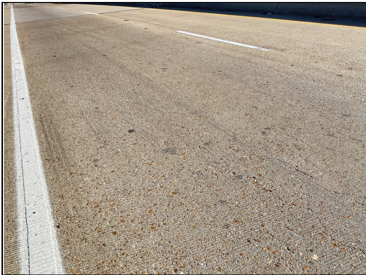
Span 1 longitudinal cracks
